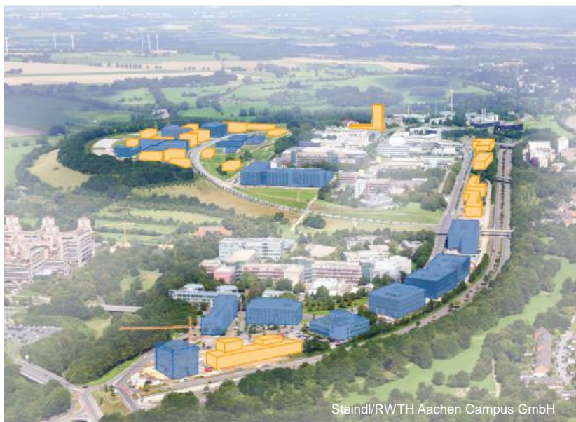
View from the South
